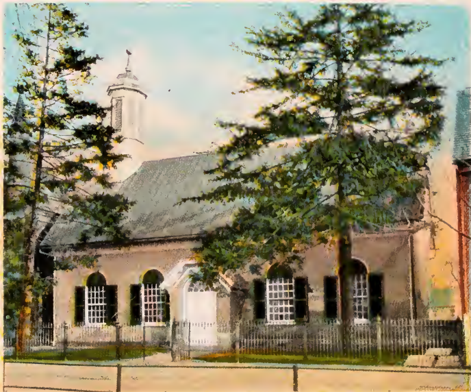
OLD CHURCH ERECTED 1707 NOW USED AS A CHURCH HOUSE
